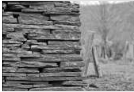
Dry-Stack Blue Stone Wall
