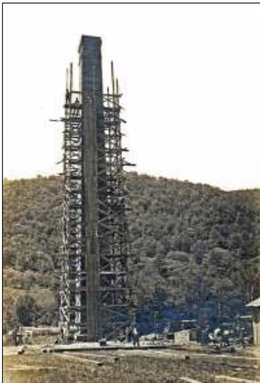
Acid Factory Chimney construction 1912
